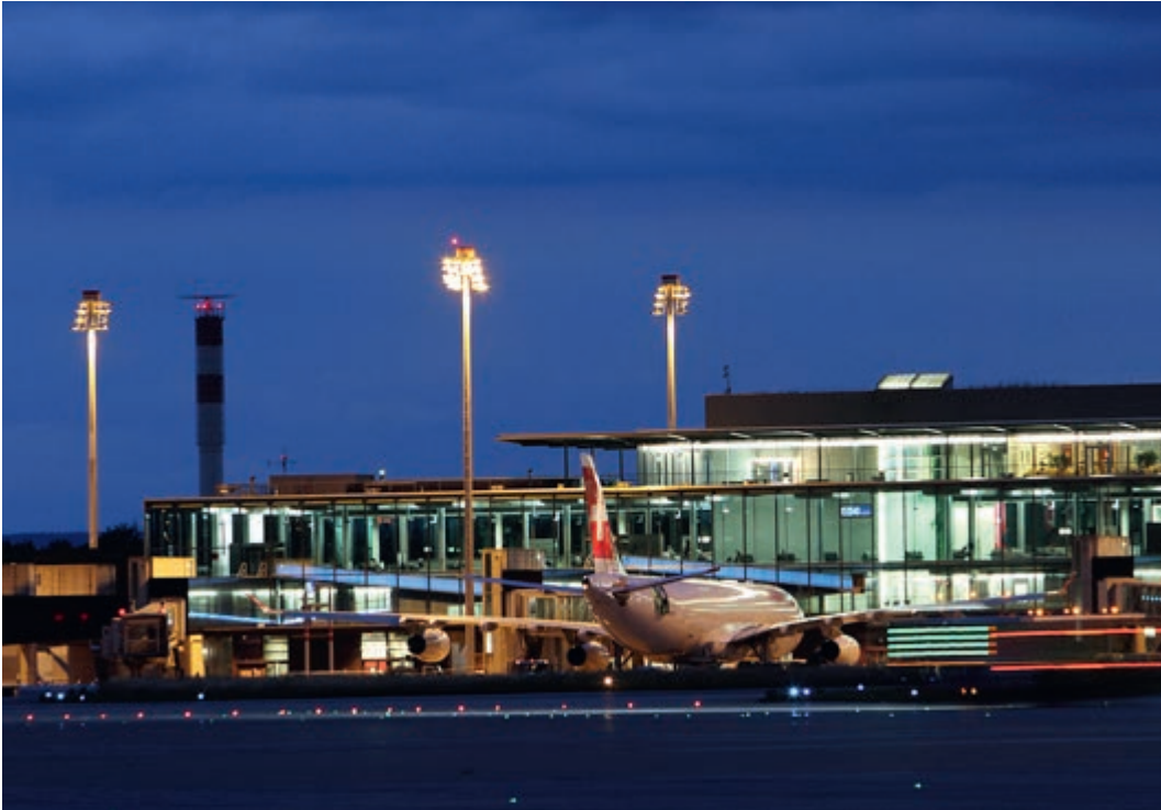
MeteoSwiss moves its headquarters from Krähbühlstrasse, Zurich to Zurich Airport.
