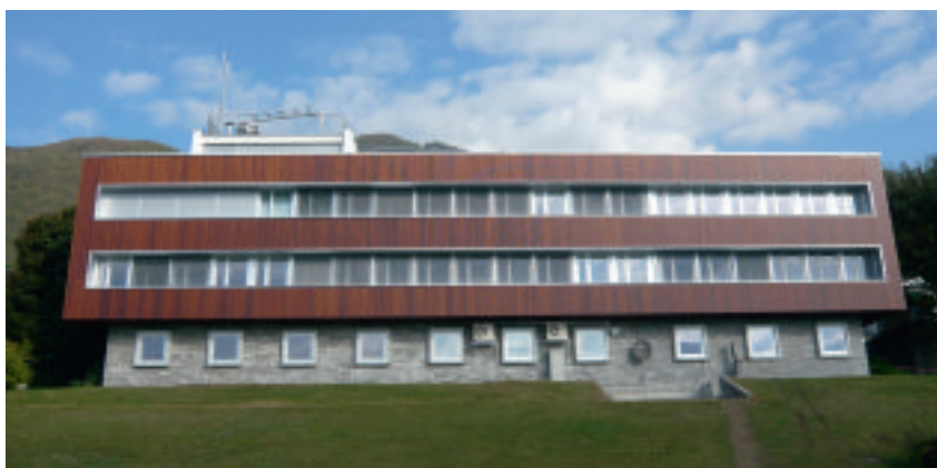
The weather centre in Locarno-Monti was renovated and now meets Minergie standards.
