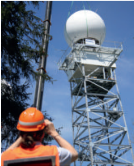
Precision work with the construction crane: Renovation of the radar on the Albis mountain in May 2012.
