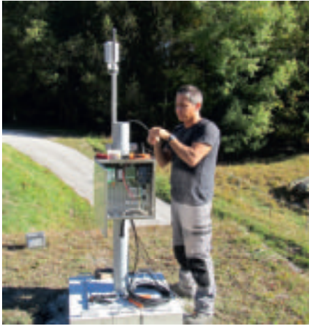
Station automation must be done manually, but then the measurements are taken automatically.
