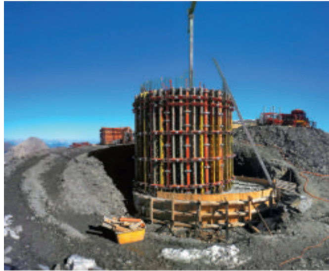
Life comes to the Plaine Morte: Construction work on the fourth Swiss weather radar started in the high mountains of the Valais in autumn 2012.
